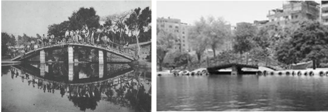
Fig.8. Original vs. current status of the wooden bridge
